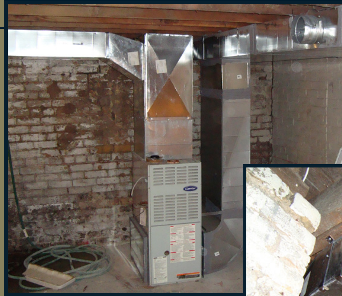
Residential construction on Pape Ave. in Toronto.
